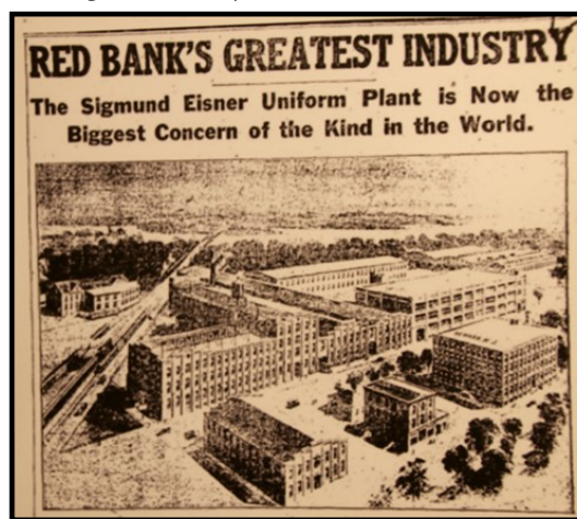
Touted in the press, the Eisner uniform manufacturing plant was a significant employer in Red Bank and other Monmouth County towns
